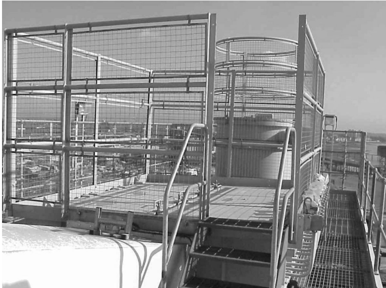
FIGURE 6-6. Top access hatch, top bag removal design
